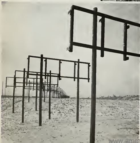
THE WIRES ON THESE POLES COMPRISE A RADIO RUNWAY FROM MANY NATIONS.
