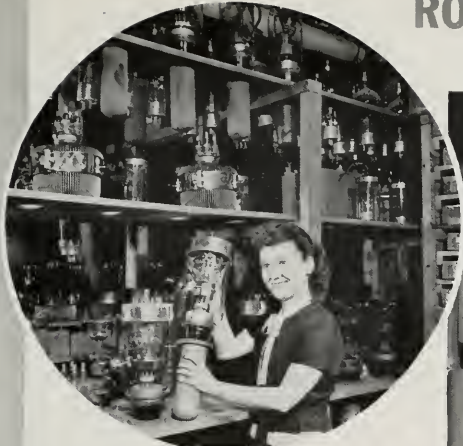
LARGE WATER-COOLED ELECTRON TUBES EMPOWER THE "VOICE" OF THE POWERFUL TRANSMITTERS AT ROCKY POINT.
